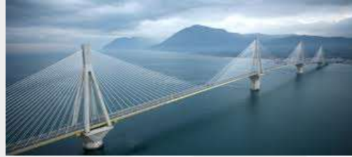
Rio – Antirio bridge
