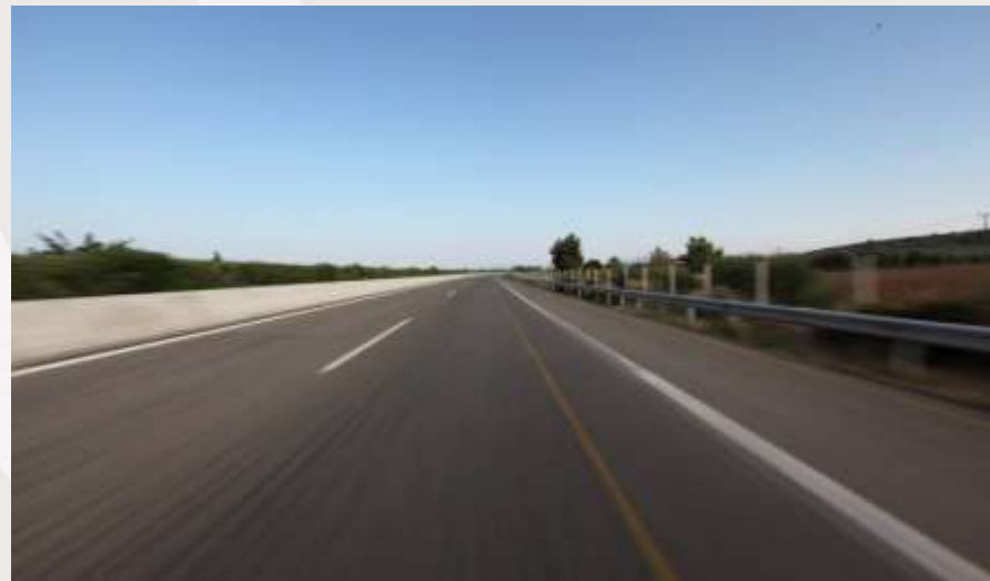
MOTORWAY OF CENTRAL GREECE
