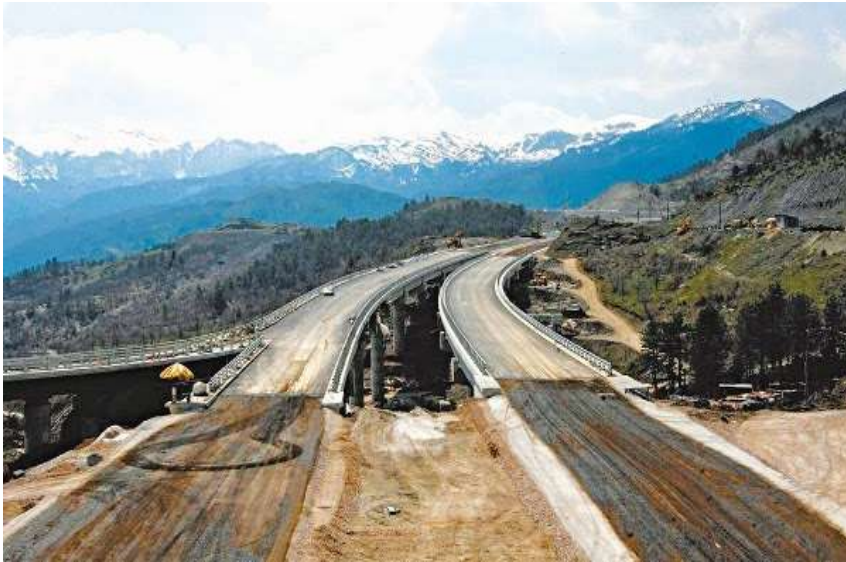
Old National Road Epirus (Initial Construction 1970)
