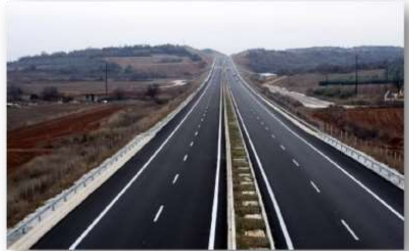
MOTORWAY OF CENTRAL GREECE
