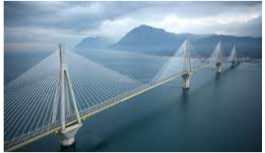
Rio – Antirio bridge
