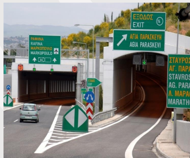
Attiki Odos (Attica Tollway)
