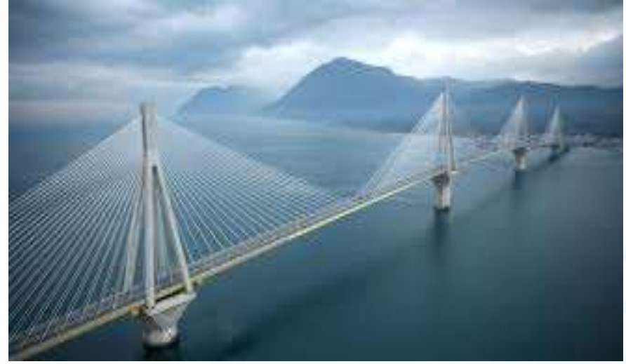
Rio – Antirio bridge
